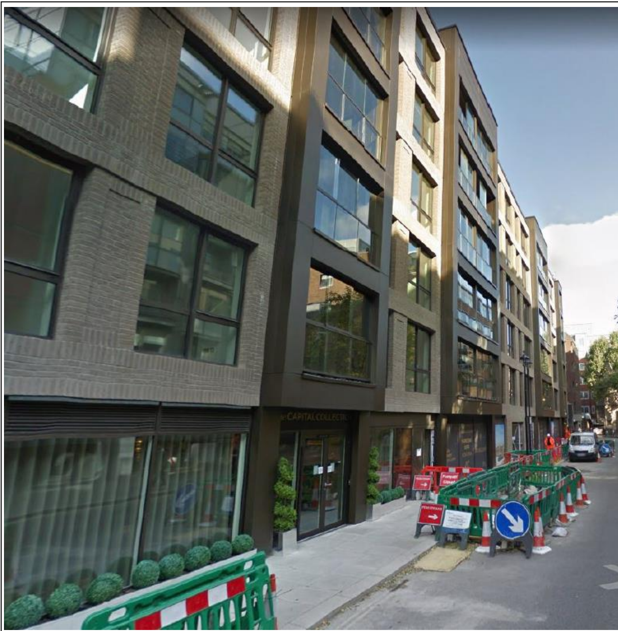
Ground floor commercial units 2 Monck Street
